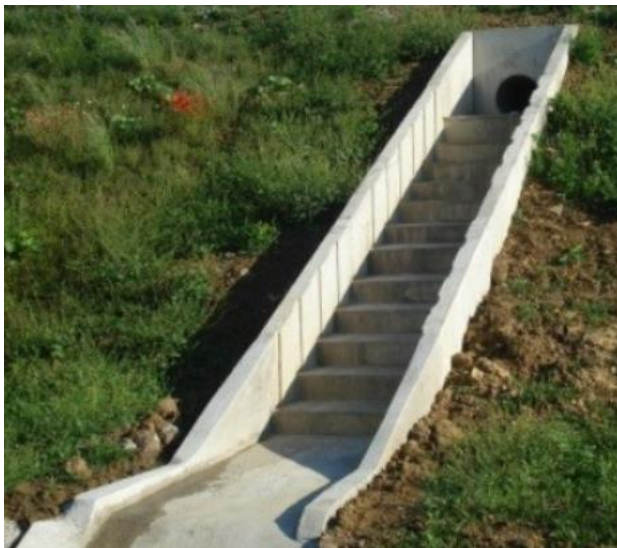
Figure 155: Staircase drainage on road embankment
