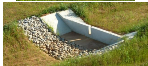
Figure 156: Cascading overflow structures in a ditch (view from downstream)
