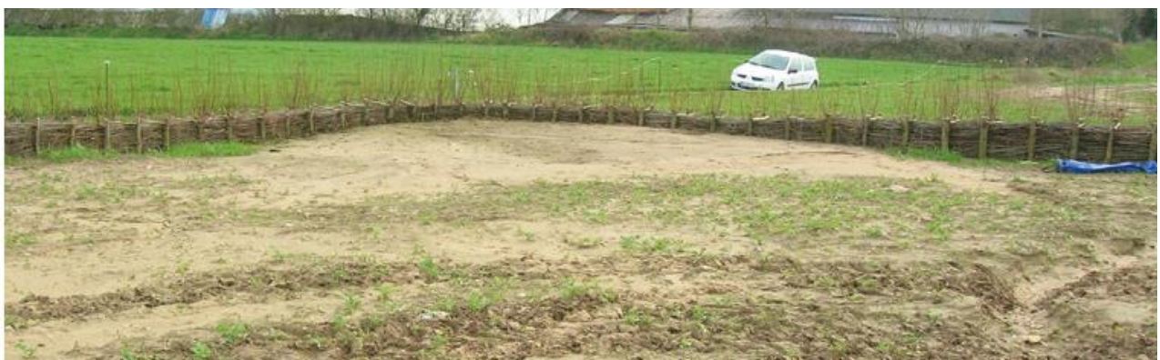
Figure 55: Sediment accumulation upstream of a fascine located at the low point of a plot subject to several gully outlets in the catchment area (France)
