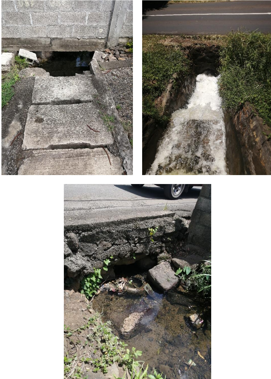
Figure 33: Inadequate Culvert Capacity
