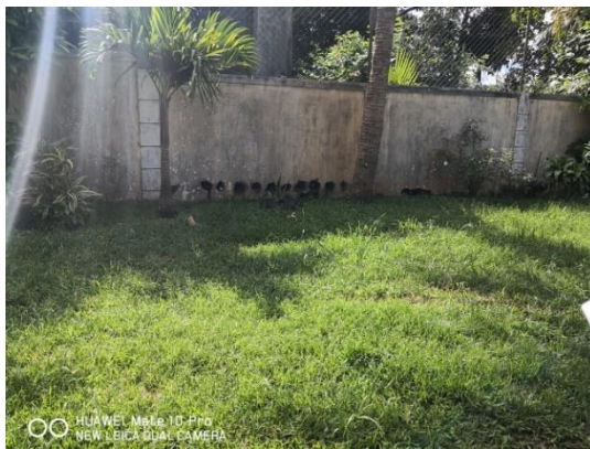
Figure 175: Holes drilled into wall to release hindered flow during flood event at Nouvelle France
