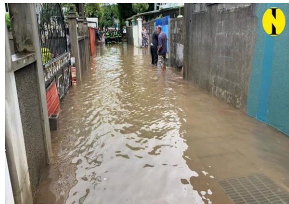
Figure 176: Boundary walls diverting flows along street and to down-slope properties at Chemin Grenier
