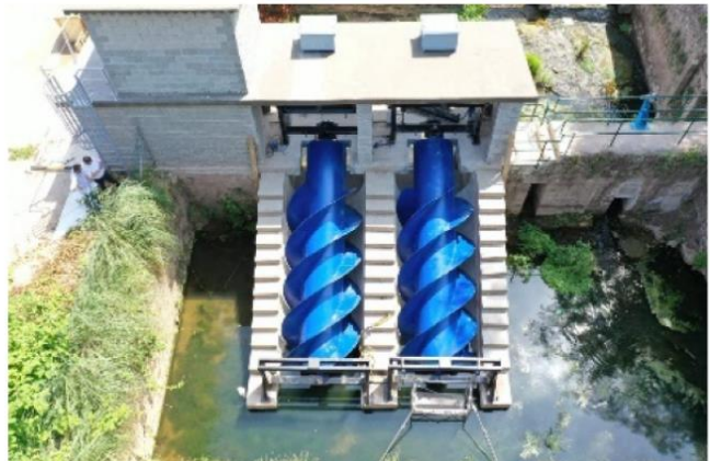
Figure 108: Pumping - Compact Archimedes screw pumps
