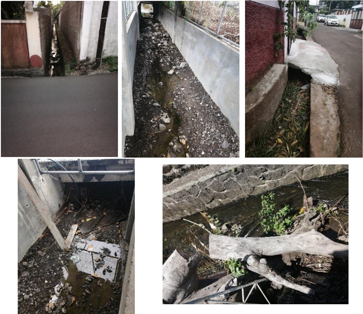
Figure 32: Poor drain network
