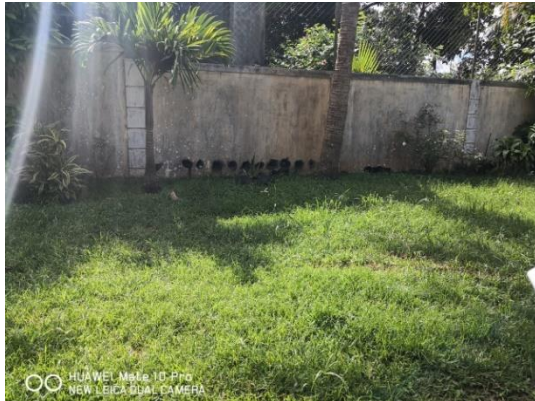
Figure 15: Holes drilled into wall to release hindered flow during flood event at Nouvelle France
