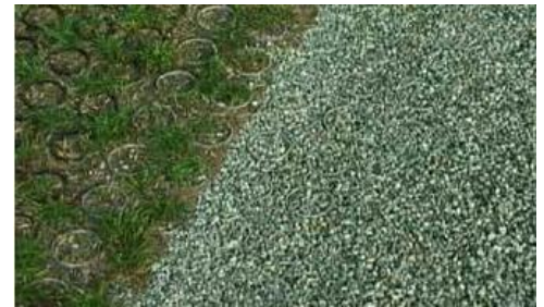
PVC mesh overlaid with soil (or grass or gravel)
