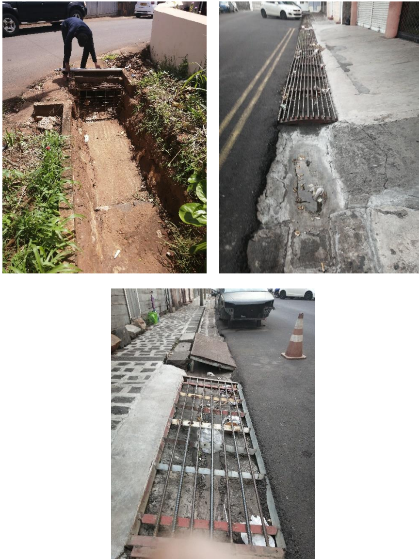
Figure 34: Insufficiency of Roadside Drains
