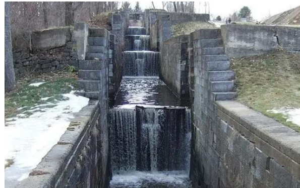
Figure 153: Stepped Canal Falls
