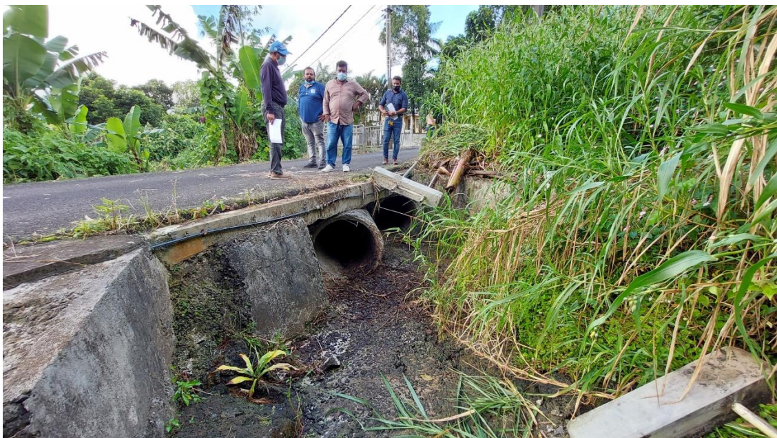
Twin 750 mm diameter concrete culvert across Nav Hind Lane
