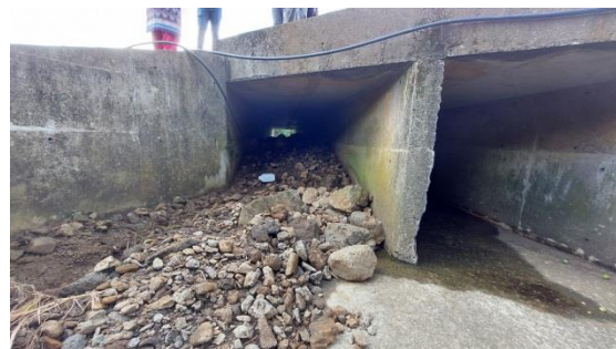
Culvert Blocked by transported rocks/sediment
