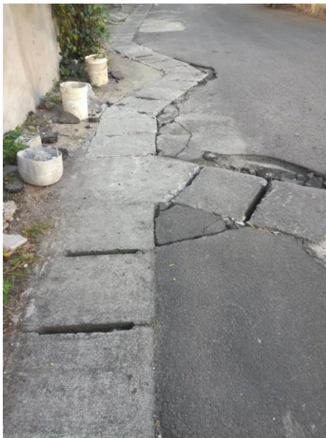
Covered RC Drain 500 mm wide x 350 mm deep
