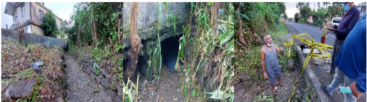
Building encroachment and diverted drain into A10 roadside drain at point W''
