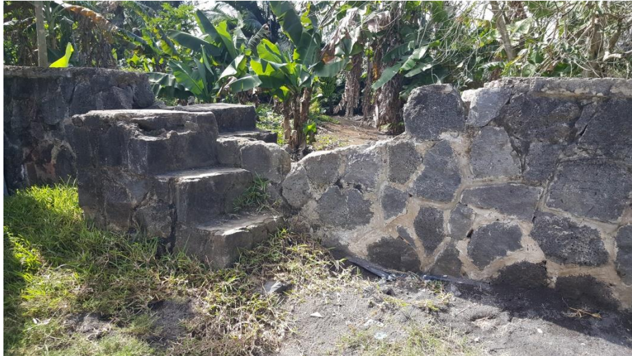
Breach into stone masonry floodwall
