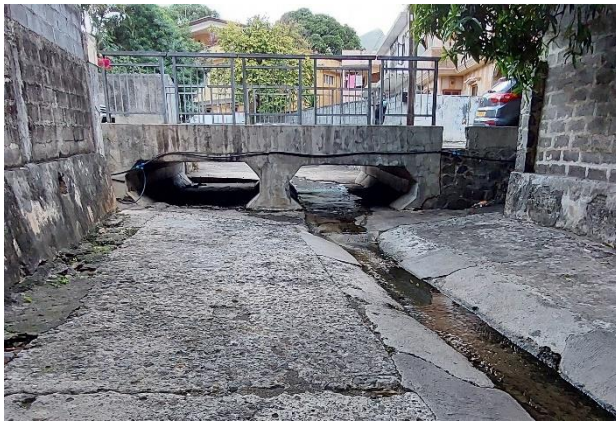
Multi-cell Culvert at Gravier Street
