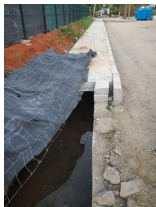
Rehabilitated drain 700 mm wide by 600 mm deep
