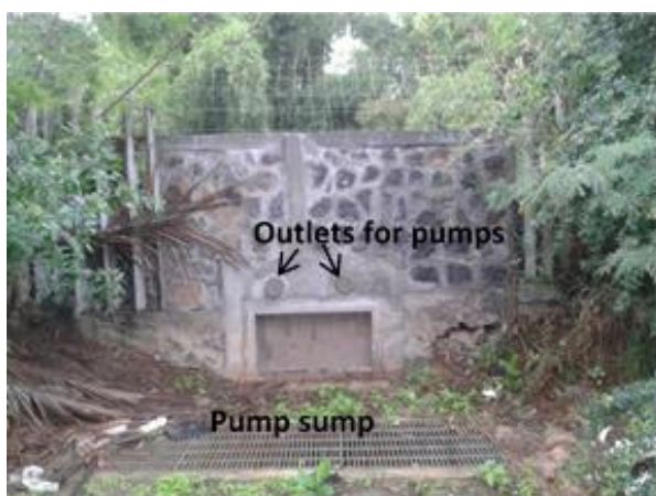
Floodwall with flap valve and pump sump
