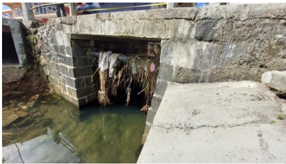
Culvert at E (note water pipe crossing)
