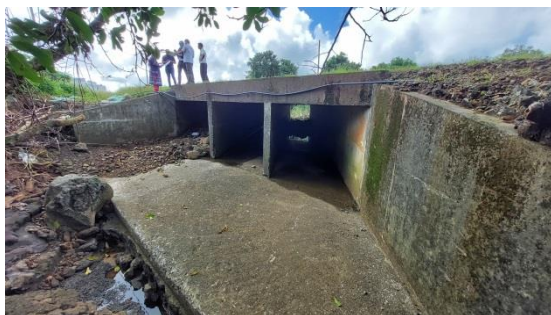
Culvert Blocked by transported rocks/sediment
