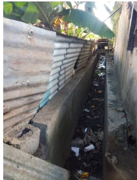
Open RC drain 470 mm wide x 450 mm deep
