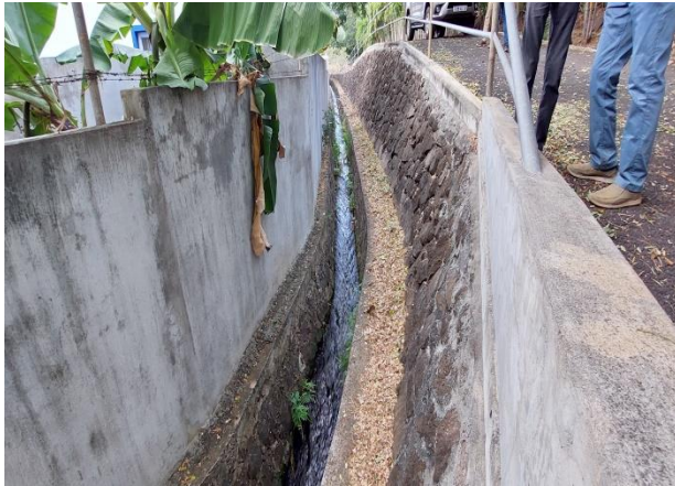
River converted into Narrow Drain and into narrower drain
