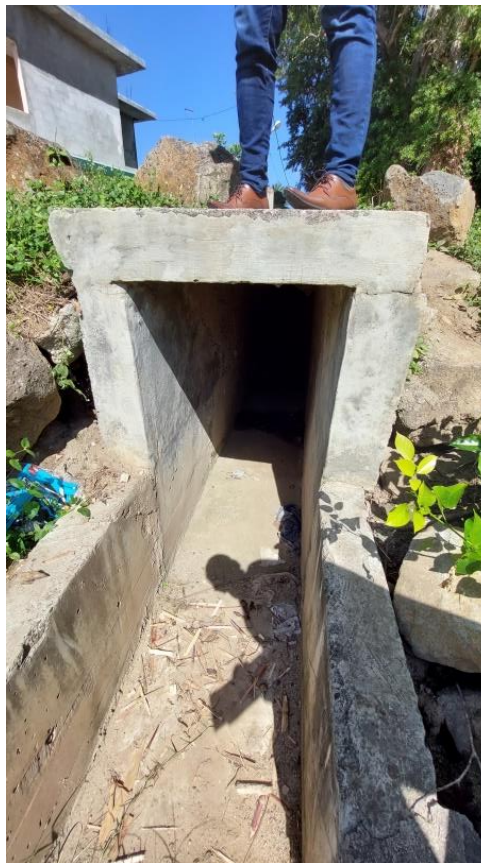
Drain Outlet 700 mm wide x 1500 mm deep into river
