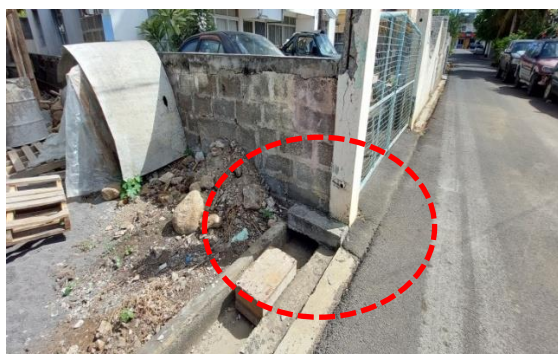
Boundary wall encroachment onto roadside drain
